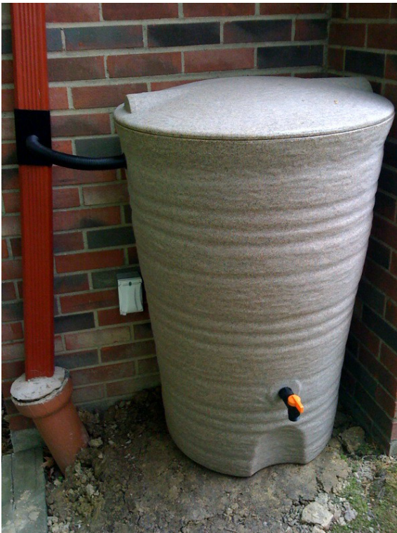
1. Example of Rain Barrel with downspout diverter that directs overflow back to the downspout
