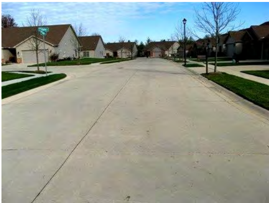
Figure 4.1. Example of concrete street in excellent condition
