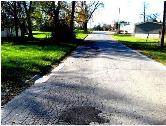
Figure 3.3. Example of asphalt street in very poor condition
