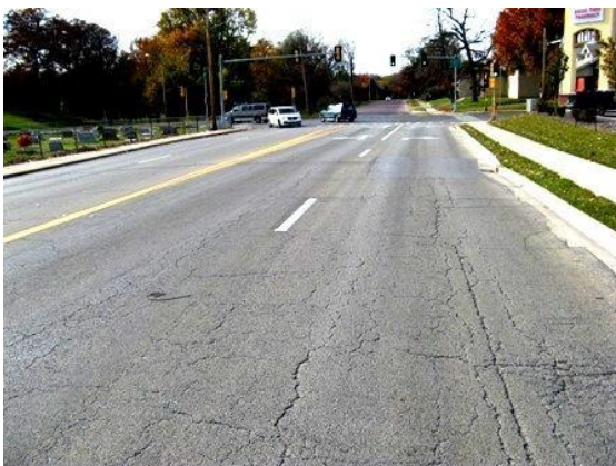
Figure 3.2. Example of asphalt street in fair condition
