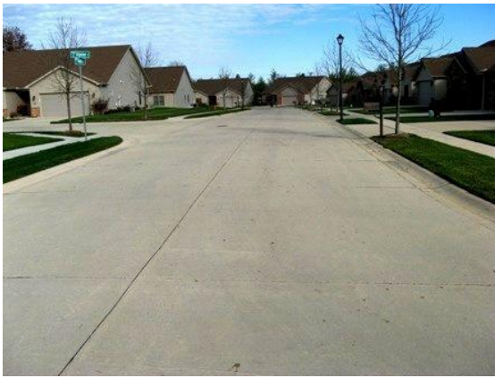
Figure 4.1. Example of concrete street in excellent condition
